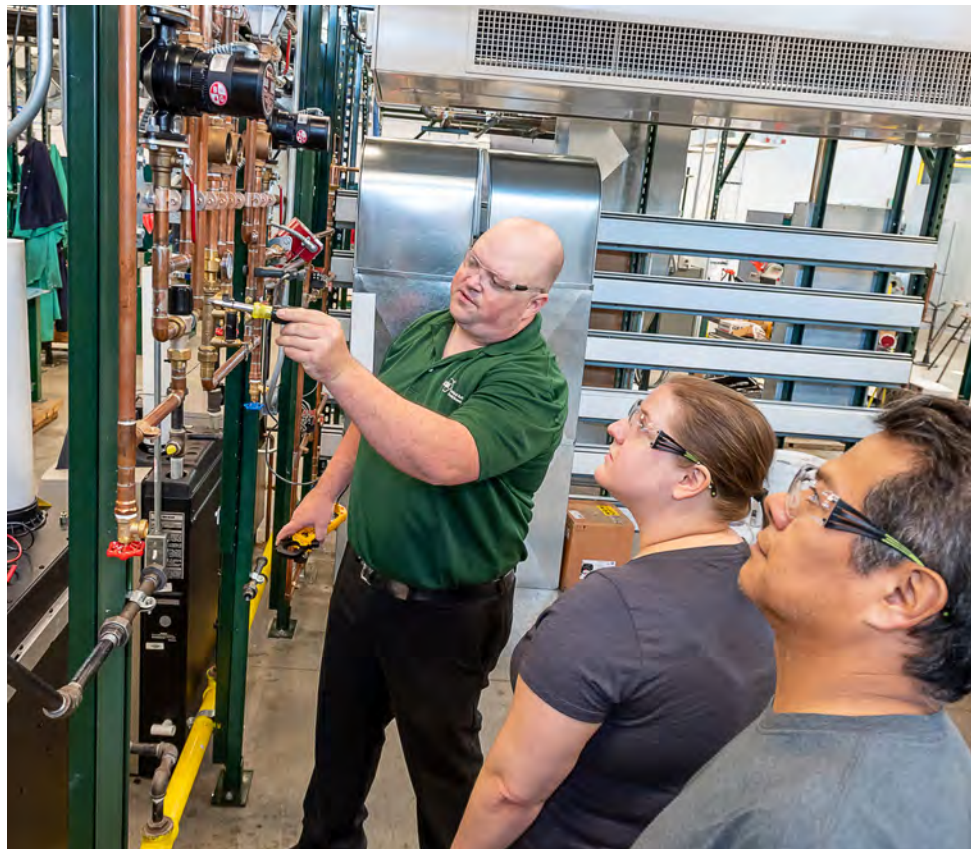
An HVAC instructor and students review hydronic balancing and mixing for radiant floor heating.
