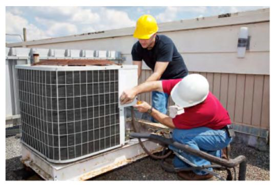
Repairing a condensing unit
