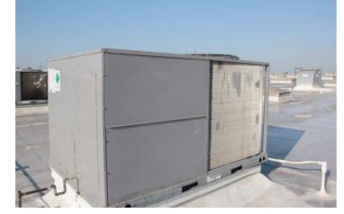
Roof mounted package AC/Heating unit
