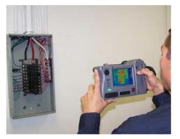
Technician using IR camera to photograph switchboard
