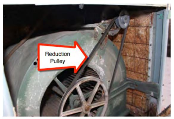
Belt drive fan with reduction pulley
