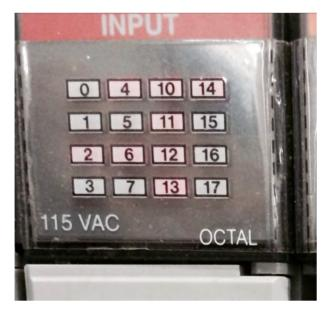
Input board indicator lights used to verify operational status
