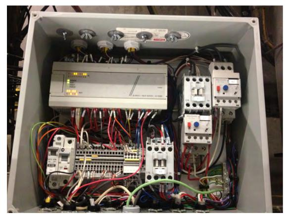
MicroLogix 1000 Controller for Combi Box machine
