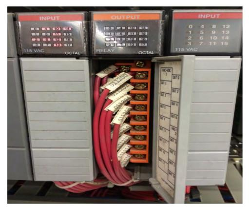
Input and Output boards for connections to a PLC, SLC 500 series
