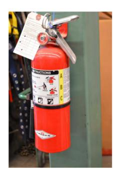
Dry chemical fire extinguisher for use on A, B or C fires. An employee may not use a fire extinguisher unless trained on its proper use by the employing company.
