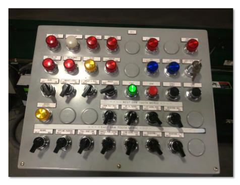
Operators' Control Station which can be used for manually switching and overriding PLC's Inputs or Outputs for operations indicated by illuminated lights
