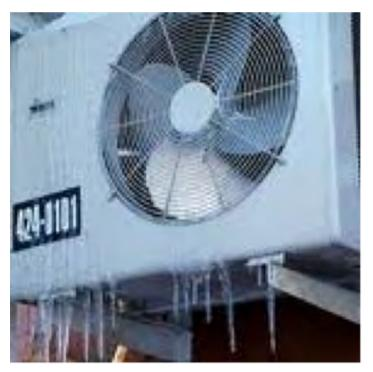
Frozen evaporator due to low temperature in the evaporator
