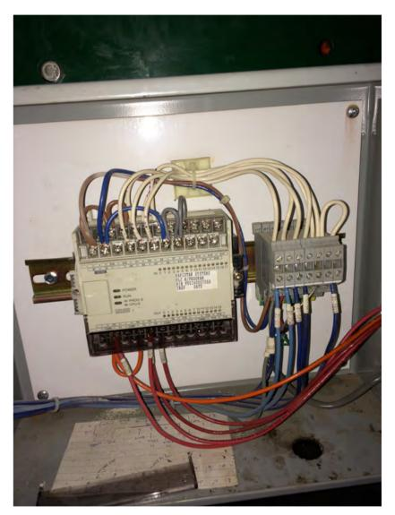
A smaller PLC made by Mitsubishi, designed to work together with an Allen Bradley PLC 5 master controller
