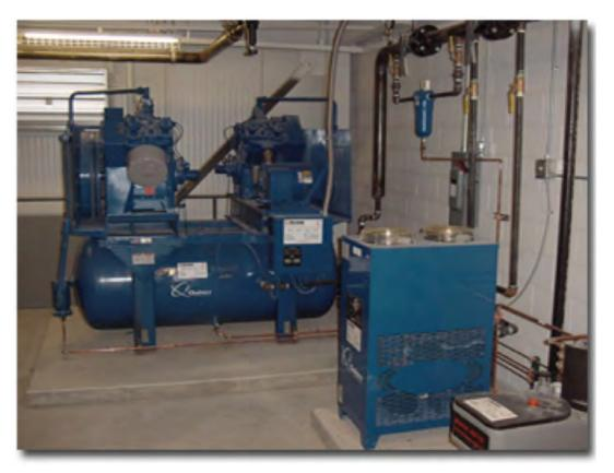
Industrial air compressor with a refrigeration drier
