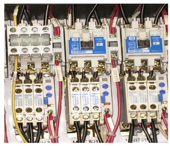
Motor starters controlled by PLC outputs that activate a relay to provide current to start a motor
