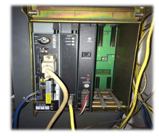
PLC 5 Master Controller with inserted EPROM, controlling the entire operation of a conveyor within a distribution center
