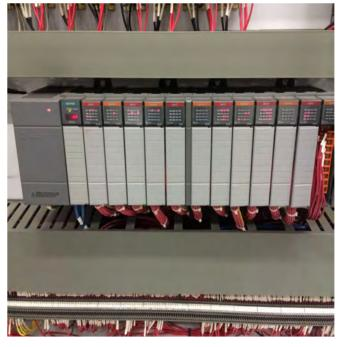
PLC rack of input and output boards
