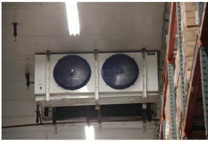
Evaporators for a commercial refrigerator
