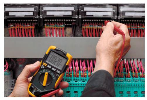
Electrical testing of low voltage control circuits
