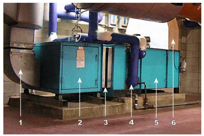
Commercial Air Handler Parts 1-Supply duct 2-Fan compartment 3-Flex connector 4-Heating and cooling coil 5-Filter area 6-Return and fresh air duct
