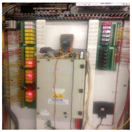
Computer controller with inputs and outputs
