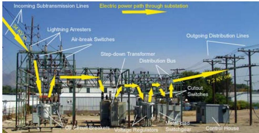
Energy flow through a typical substation
