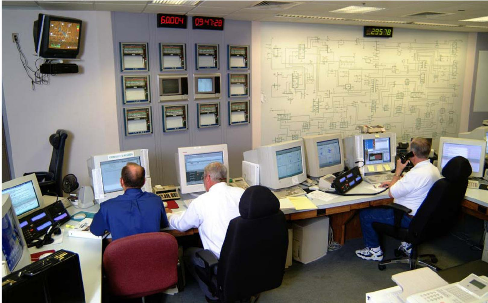
**Figure 4.3.** This photo highlights the key features of a control center. On the far right is a map. Although it is too small to show these details, the map indicates the location of power plants and transmission lines under the control of the center, usually with colored lights that indicate the status of the power plant or transmission line (e.g., red for out of service). Connections to adjacent control areas are also indicated.
