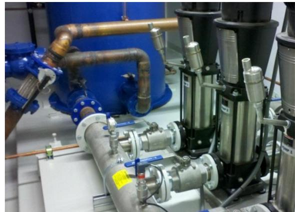
**Figure 4: Domestic water pressure station**
