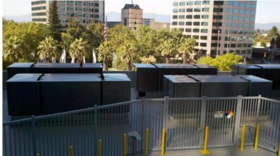
**Figure 16: Fuel cells on roof at Adobe Systems**
