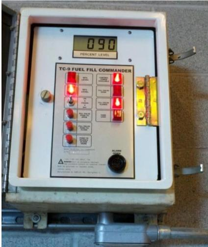
**Figure 1: Enclosure with generator fuel indicators**
