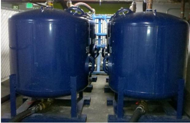
**Figure 6: Carbon filters used to treat groundwater**
