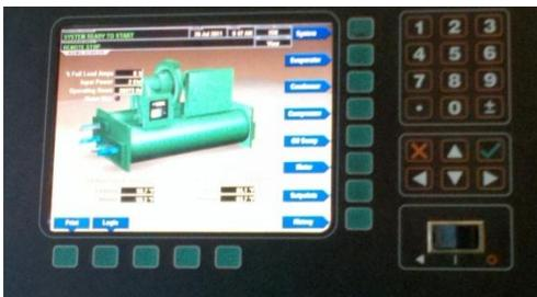
**Figure 3: Chiller control panel**
