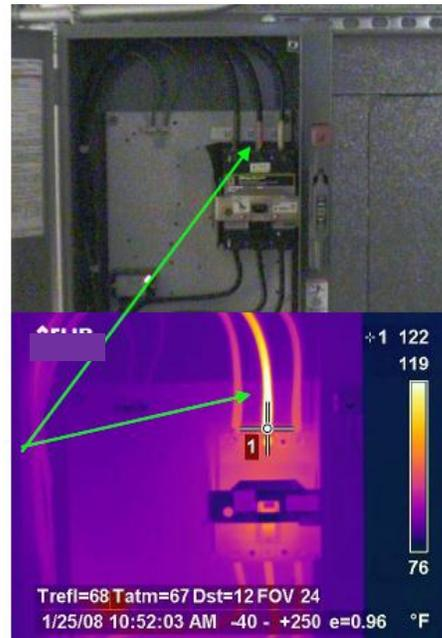
**Figure 6: Image seen through an infrared camera of a hot spot on a motor starter control breaker**
